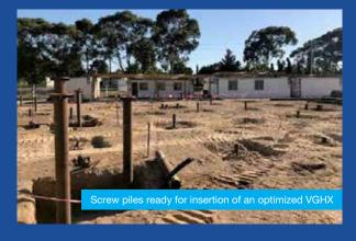
The GSHP system integrates the thermal heat loops within the structural screw piles for geothermal heat exchange, achieving the required heat transfer by utilizing the vertical steel piles required for structural footings.
